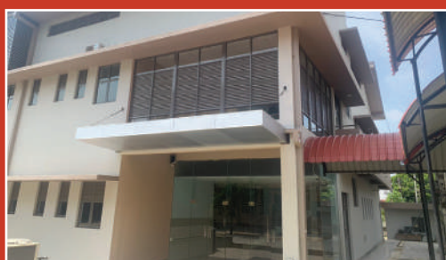
Construction of Surgical unit in Teaching Hospital, Batticaloa for SLR 302 million
